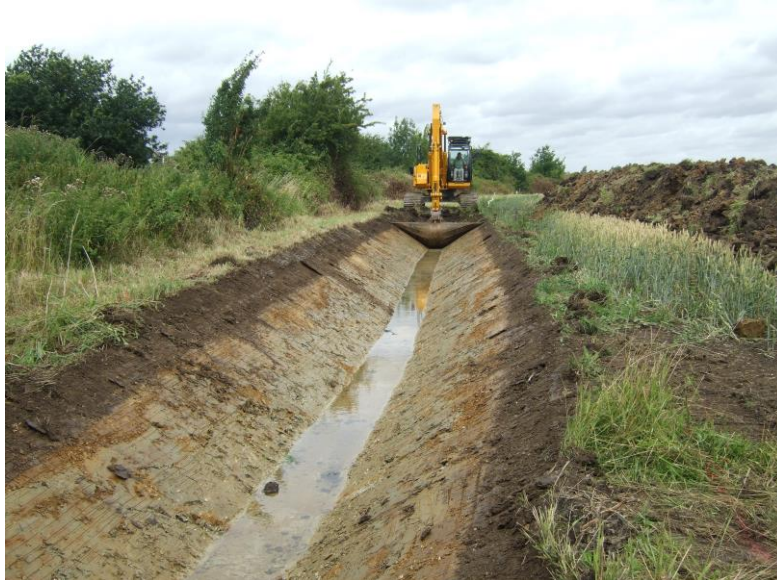
Figure 10-1: Completed action to create a new ditch near Eye Green to reduce flooding
