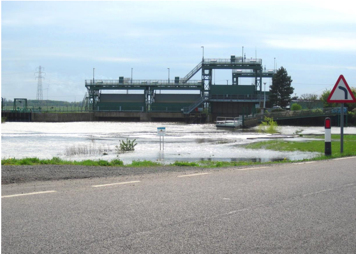
Figure 7-2: Dog in the Doublet sluice during a very high tide. Source: Peterborough City Council
